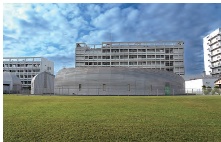
▼ The facade of the Central NMR Complex is visible in the foreground. Behind it is the Central Research Building, to which a covered walkway connects it.
