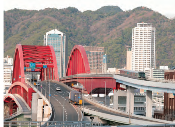
▲ The Portopia Bridge (right) running parallel to the Kobe Bridge (left) is a bridge specifically for the Port Liner train operated by Kobe New Transit.
